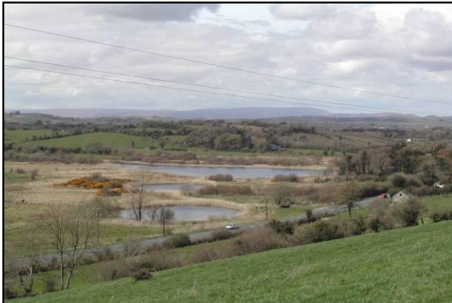
Plate 5 Ardloy and Aghalenane Loughs with the existing N4 in the foreground.
